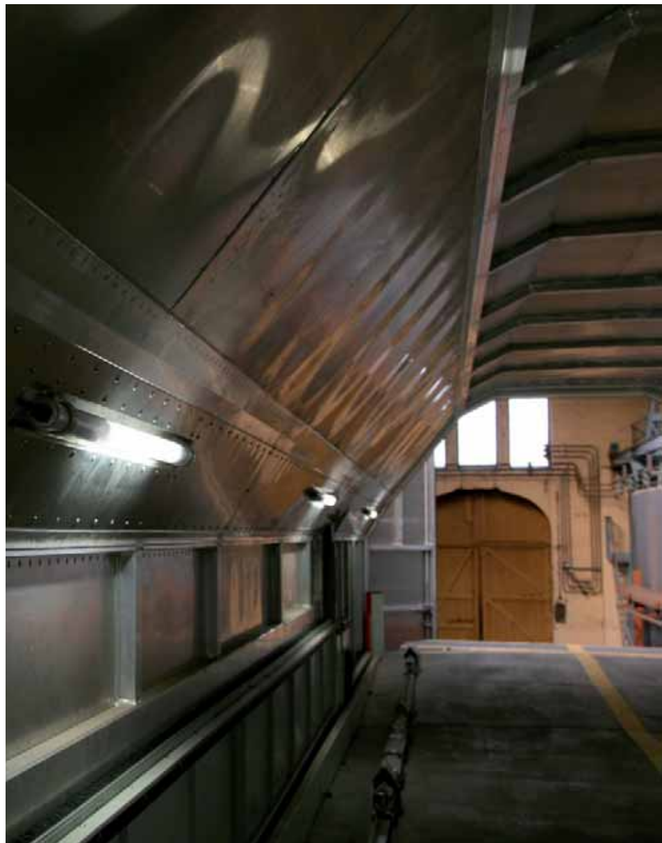
LUZERN 38 LED tubular luminaire, 24 V DC, 80 lm/W, beam angle 120°, 5400 K, PMMA tube, transopal
